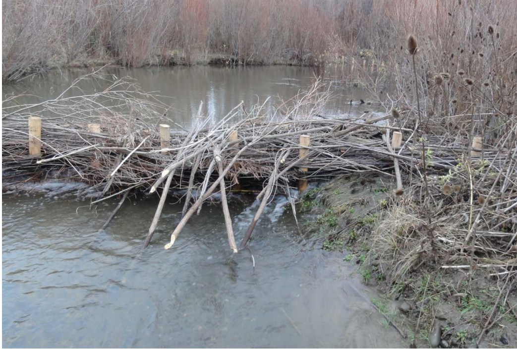
Figure 11. A PLWW is similar to an SD, but acts more like a weir in that water is allowed to flow through the willow branches such that low flows are not overtopping the structure and the woven branches may not extend to the top of the posts. These may naturally seal up by trapping sediment and organic material moving downstream or they may be utilized by beaver. Note that beaver have started to colonize this PLWW, as evidenced by the chewed stems aligned parallel to the flow in the middle of the photograph.
