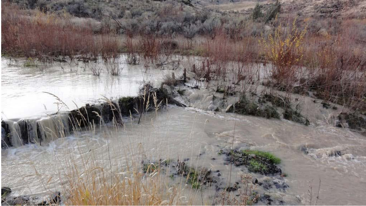
Figure 10. A typical SD (SF-17 at Sunflower) with willow branches woven between vertical posts and the back side sealed with rock and clay. Note that the dam height is sufficient to divert flow onto the river left terrace, mimicking a stable beaver dam.
