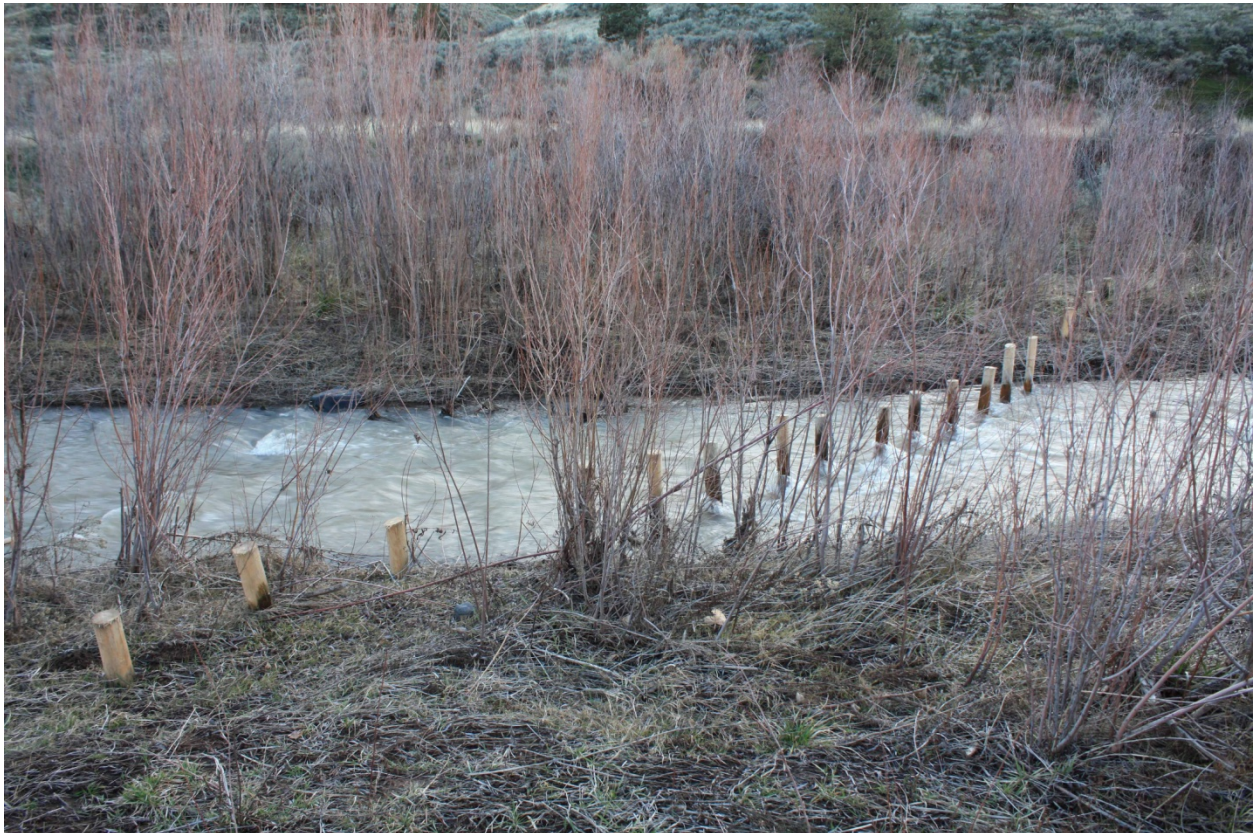
Figure 12. The purpose of a PL is to provide a site where beaver can build a stable dam. They generally create little or no geomorphic changes unless utilized by beaver.
