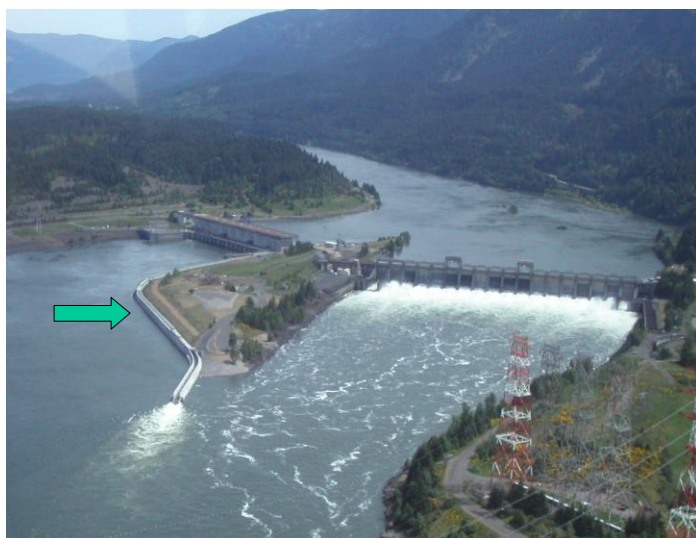
Figure 1. Aerial photo of Bonneville Dam taken by the U.S. Army Corps of Engineers. The arrow points to the straight section of the exit flume for the new corner-collector bypass system where the PIT-tag antenna was installed (the photo was taken before it was installed).
