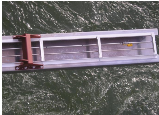
Figure 13. Top: Collector assembly being lowered into place. Note the steel beam attached to the distal end of the collector, which was used to hold the whole assembly in place. Bottom: Collector ramp prior to submersion showing the camera used to position it on the transition structure.
