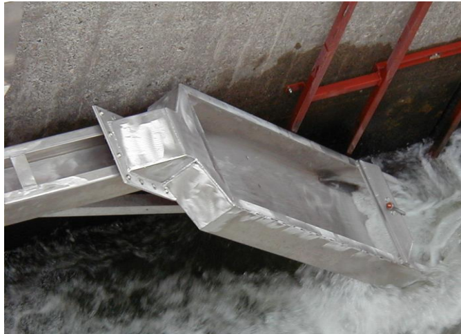
Figure 4. Photo of the Bradford Island LPS collector. Note the lamprey that is moving up the ramp near the water surface.
