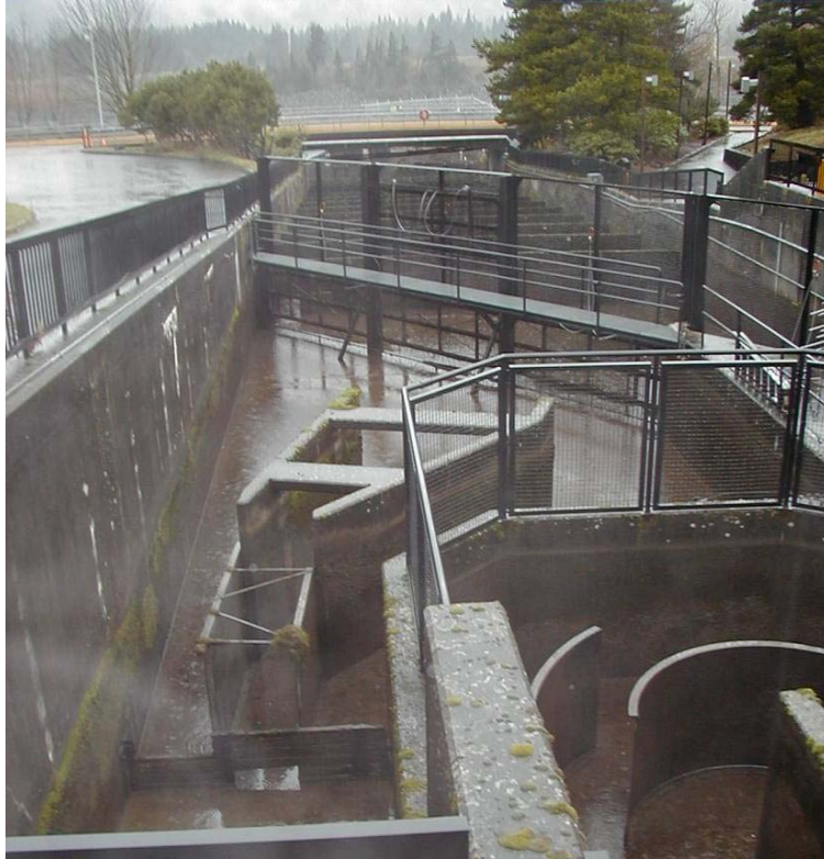
Figure 19. View looking downstream to the picket lead at the dewatered Bradford Island Auxiliary Water Supply channel. The west wall of the channel is located on the left in this photo.
