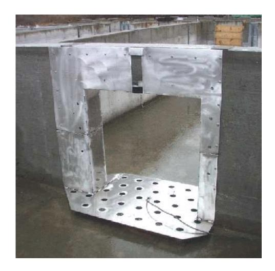
Figure 2. Photo of the alternate continuous RF shield (note welded strip at the top of the shield) that will be installed into the fish ladders during FY01. When shields are installed at the dams, the floor sections will be 8 inches beneath the fish ladder floor (not flush with the floor as shown in the photo).
