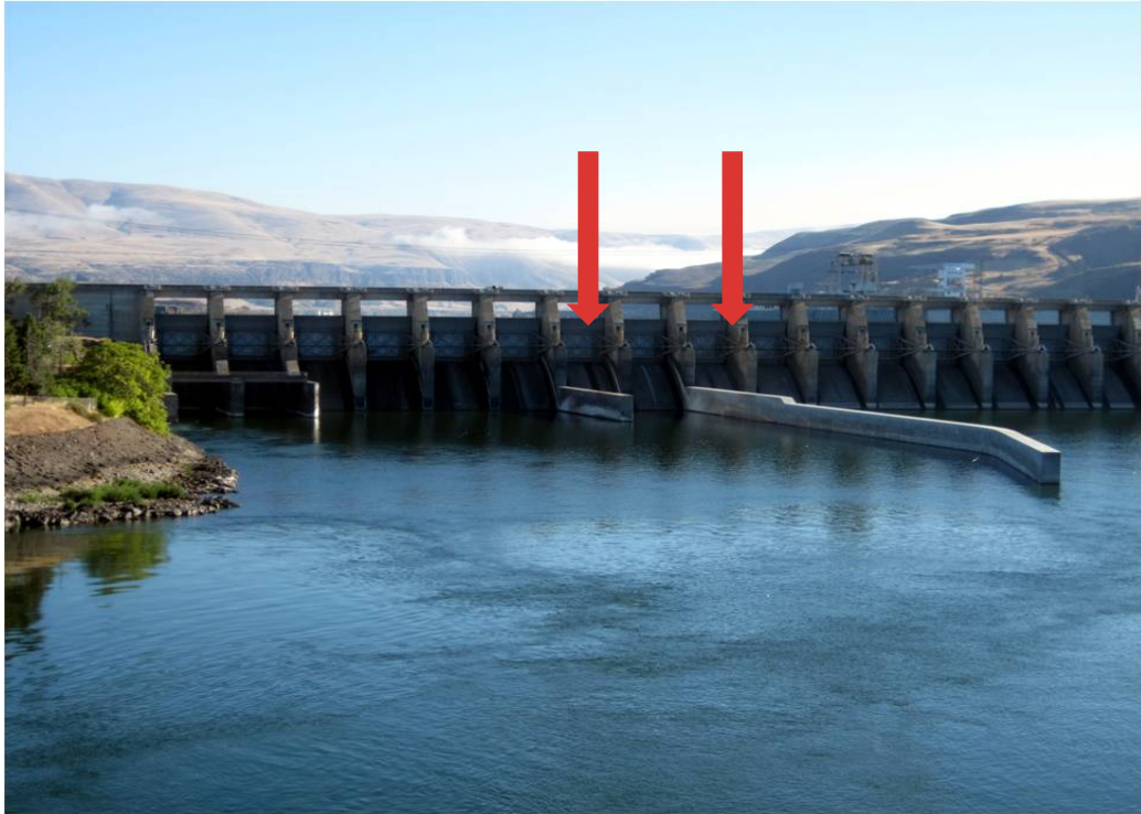
Figure 1. Photograph of spill walls at bays 6-7 (left arrow) and 8-9 (right arrow) at The Dalles Dam in 2010.
