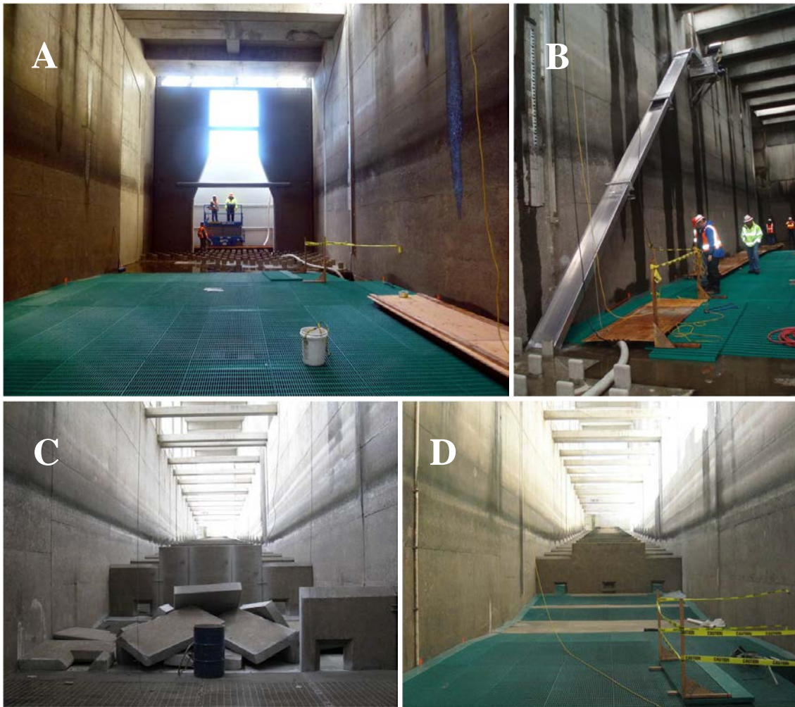
Figure 15. Modifications to the John Day Dam north fishway entrance area; camera is facing upstream in all photos except A. From left to right, clockwise: A) downstream variable-width entrance weir, bollard field, and closed entrance slot (new concrete on left wall); B) lamprey passage structure (with bollard field in foreground); C) removal of concrete weirs; and D) completed fishway with concrete weirs removed.
