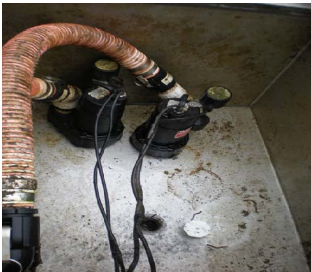
Figure C7. Upstream transition pond showing pumps and unplugged drain in reservoir at Cascades Island LPS.
