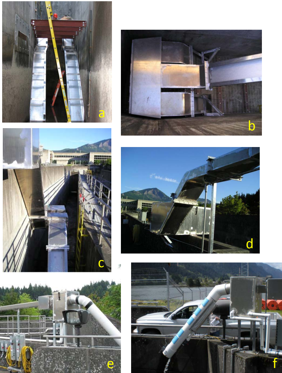
Figure A3. Photos of Washington Shore lamprey passage structure showing ramps converging at Rest Box 1 (a), Rest Box 1 (b), switchback at Rest Box 2 (c), Rest Box 3 (d), upwelling box (e), and exit slide (f).
