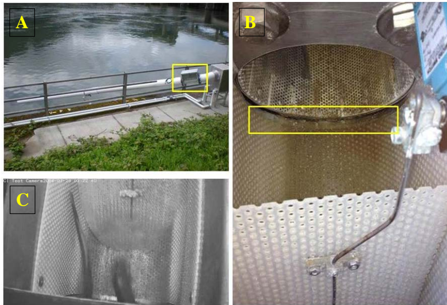
Figure 25. Photos of the Cascades Island LPS exit (A, yellow outline), the gap in perforated plate (B, yellow outline), and lamprey passing under the counter paddle (C).
