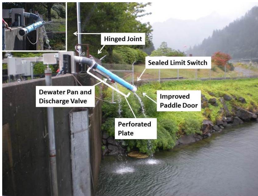
Figure 7. Photograph of redesigned exit slide at Bradford Island AWS LPS with features labeled.
