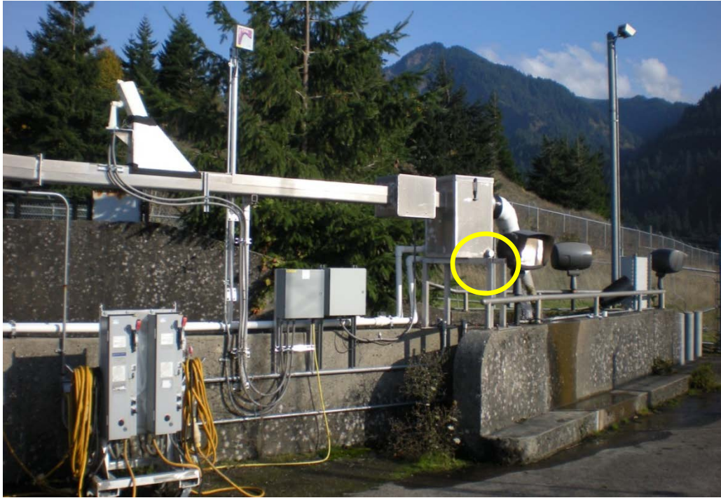
Figure A4. Discharge valve at Washington Shore AWS LPS upwelling box.
